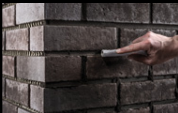
Jointing with a trowel allows you to create different looks.
